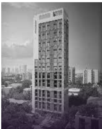
SEERVAI BUILDING GRANT ROAD, TARDEO
